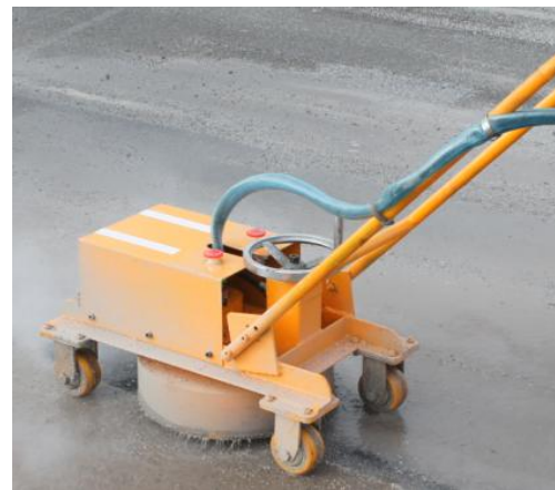
Pavement hot melt paint cleaning
